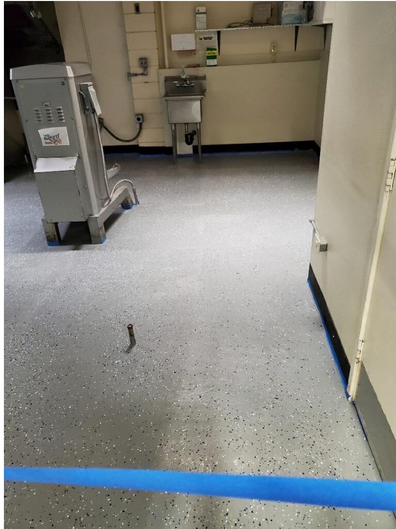
Lone Tree Kitchen – New Floor w/Epoxy Paint
